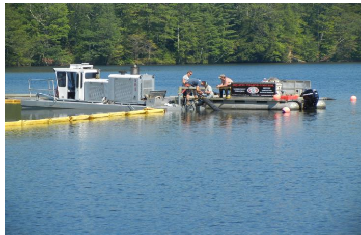
The dredger at work in Round Pond
