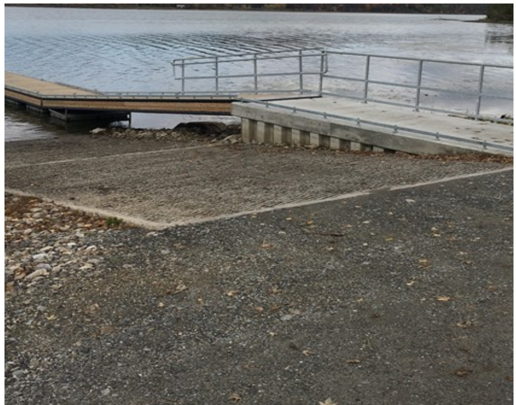
Figure C.2. Benson Landing, dock and ramp
