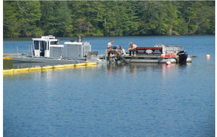
The dredger at work in Round Pond
