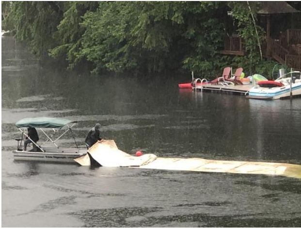
Bottom barriers being deployed in Round Pond
